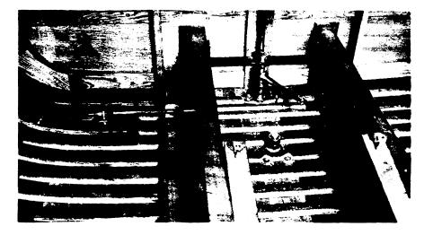
Fig. 15 Typical Bed, Stringer and Steering Set-up
